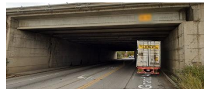
Grand Avenue Underpass of I-294.
