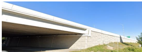
Touhy Avenue Overpass and Retaining Wall
