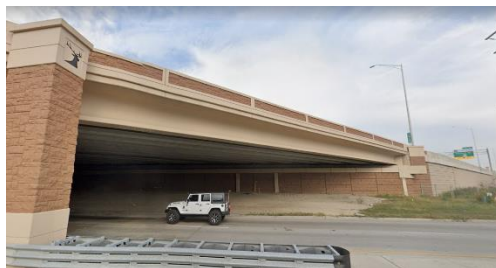
Busse Road Overpass and Retaining Wall
