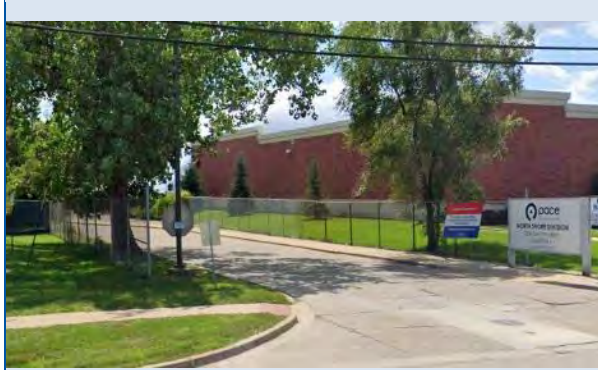
Representative Inspection Photo
