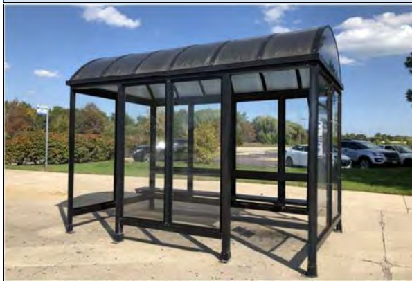
Representative Inspection Photo
