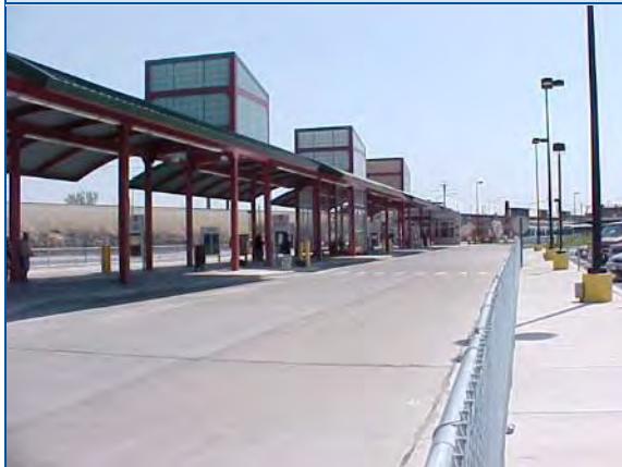
Representative Inspection Photo
