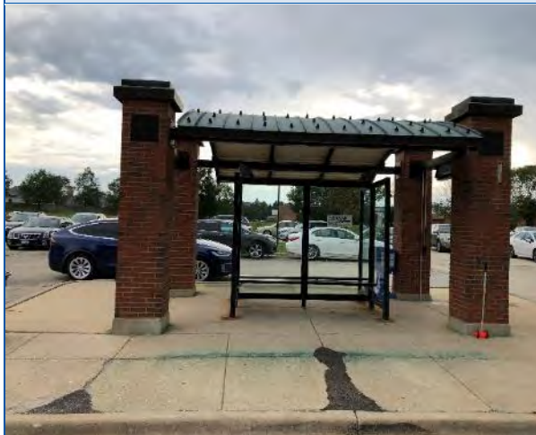
Representative Inspection Photo
