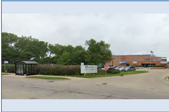
Representative Inspection Photo
