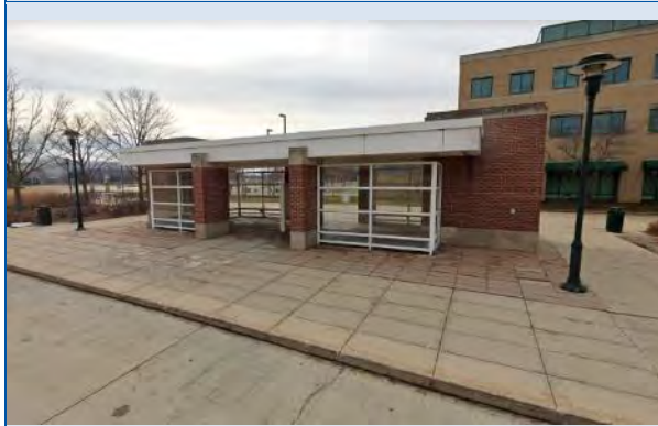
Representative Inspection Photo
