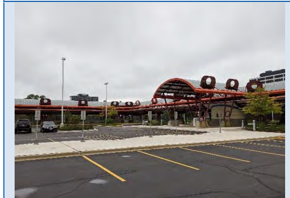
Representative Inspection Photo
