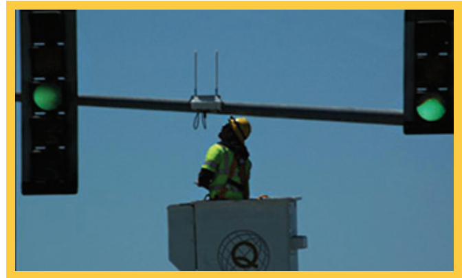
TSP allows bus transit vehicles to adhere to their published schedule by giving priority green time to buses that are behind schedule.
