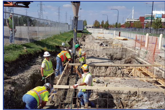
Work on the future passenger facility at Toyota Park in Bridgeview will be completed in 2019.
