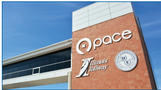
Pace partnered with the Illinois Tollway to construct a pedestrian bridge over I-90 to allow commuters access to both eastbound and westbound buses.
