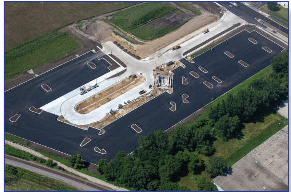
The parking lot at the new Plainfield Park-n-Ride is now operational, providing additional parking for the I-55 Bus On Shoulder service.
