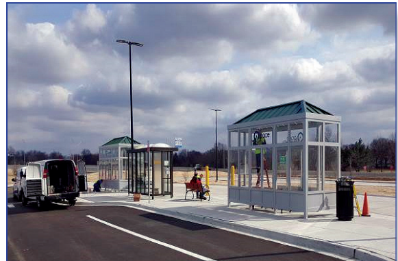
Heated bus shelters were installed at the new I-25 Park-n-Ride, which supports the Bus On Shoulder service on I-90.
