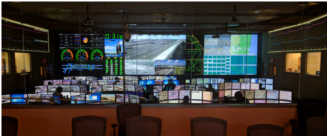
One of Florida Department of Transportation's Regional Transportation Management Centers ( www.fdot.gov ).
