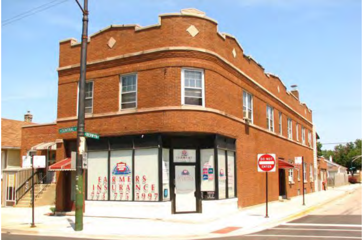
Building 026 - 5301 N. Central Avenue
