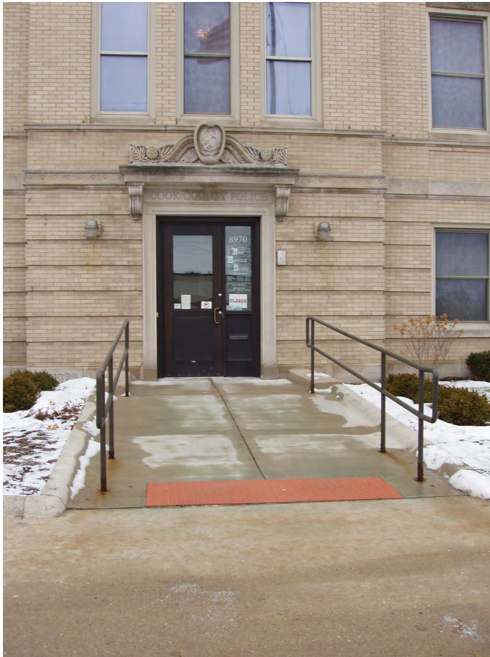
Doorway of Cook County Sheriff Building (Building 009)
