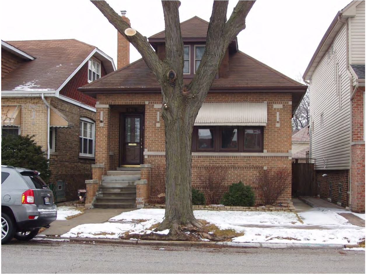
Building 023 - 5841 N. Austin Avenue
