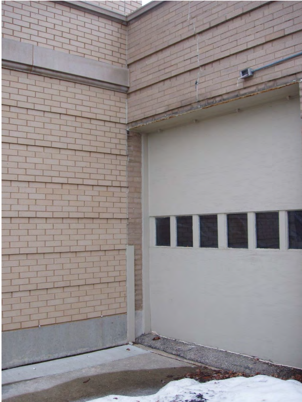
Building Seam on 8970 N. Milwaukee Avenue (Building 009)
