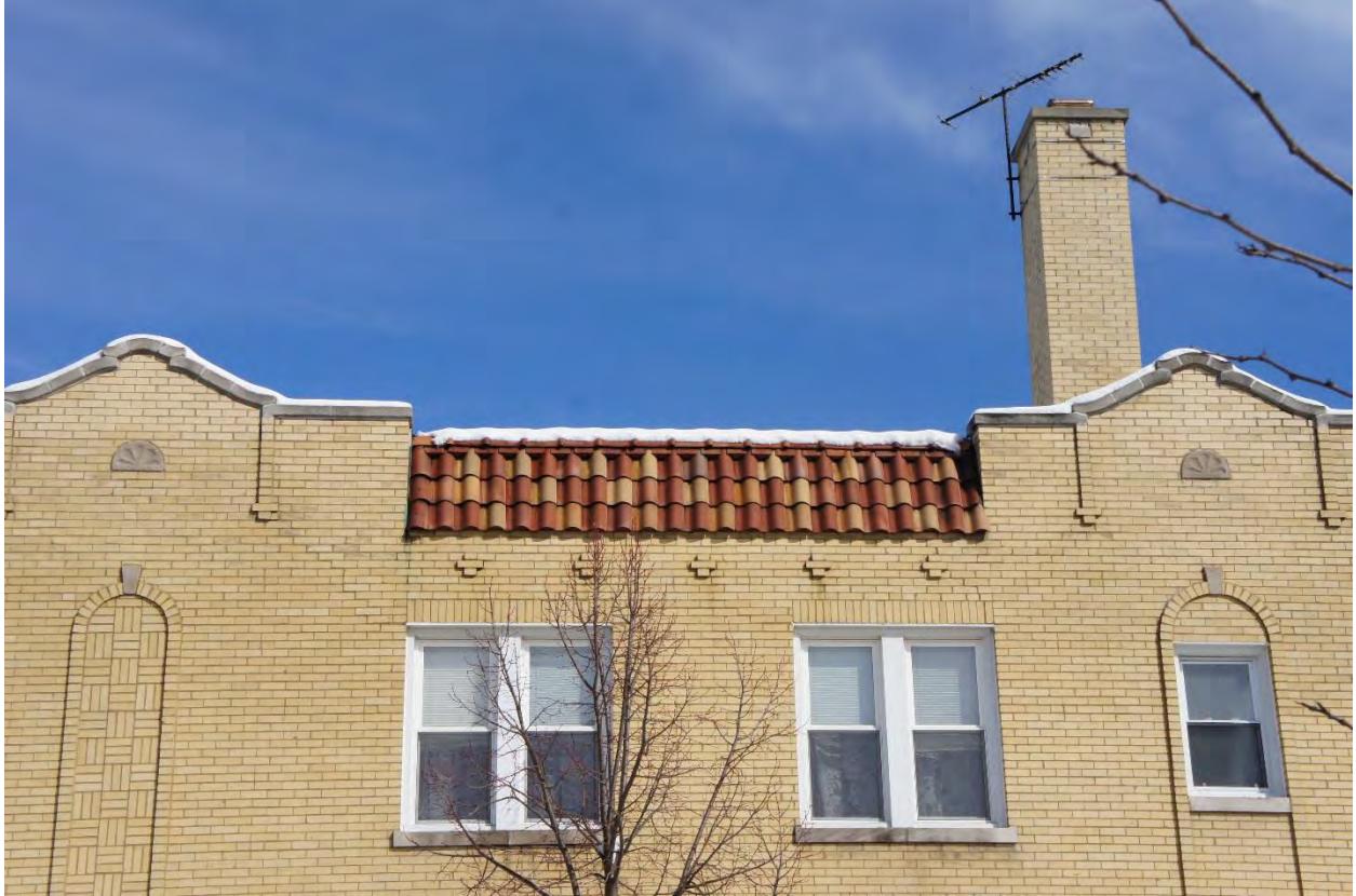
View of Roof Tiling Building 027- 5802 N. Mason Avenue
