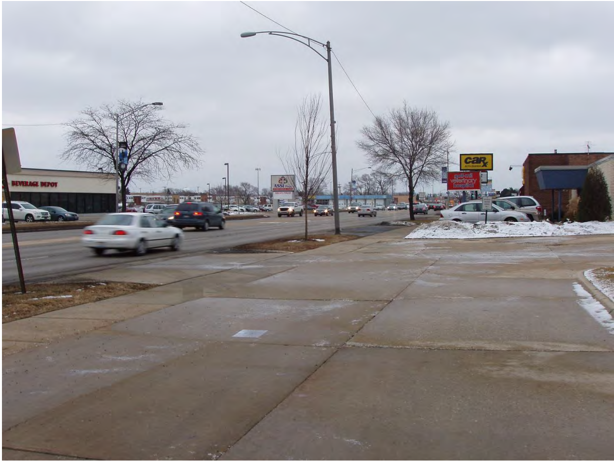
View to South from 8970 N. Milwaukee Avenue (Building 009)
