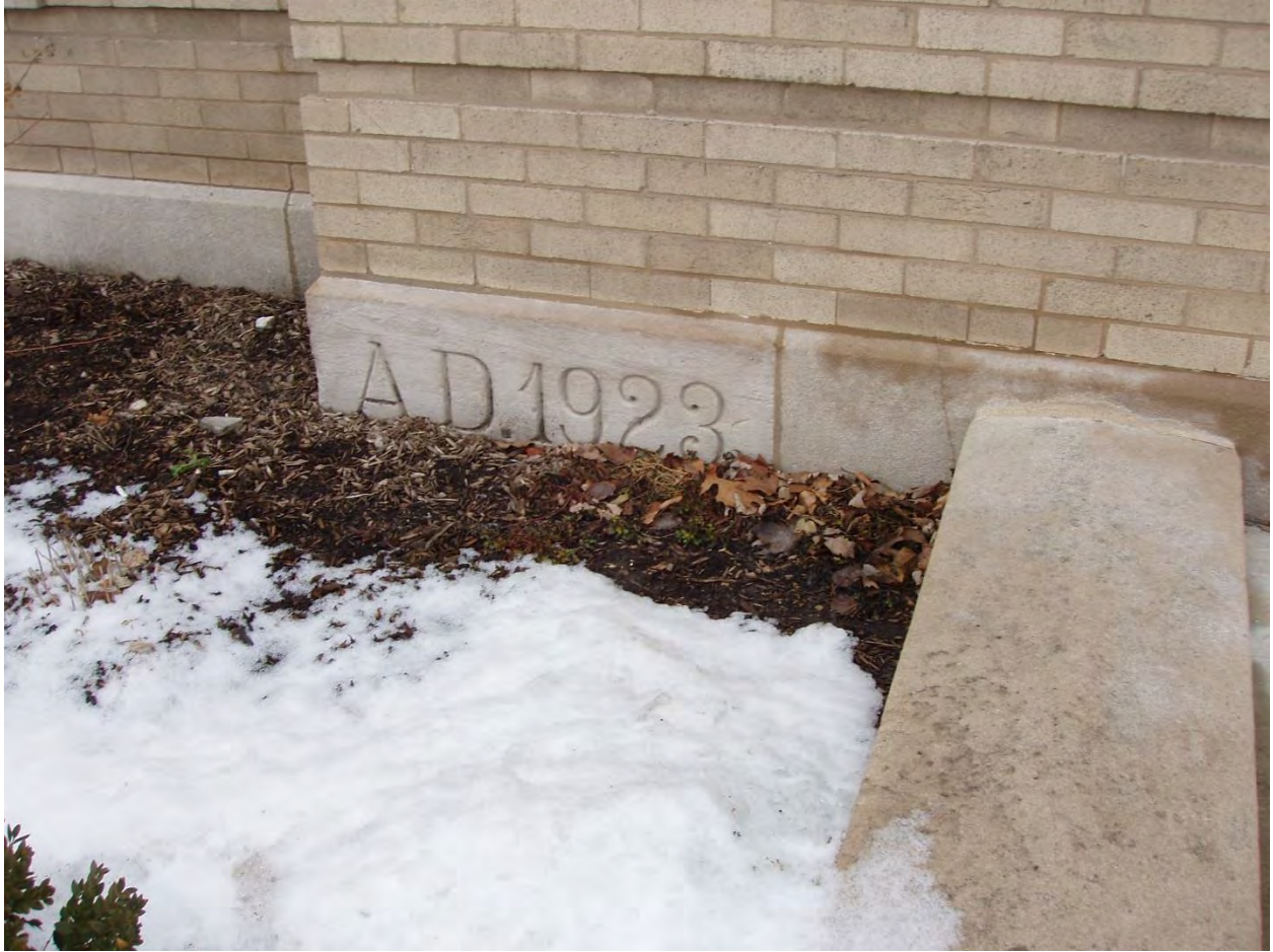
Building 009 - Foundation Stone (AD 1923)
