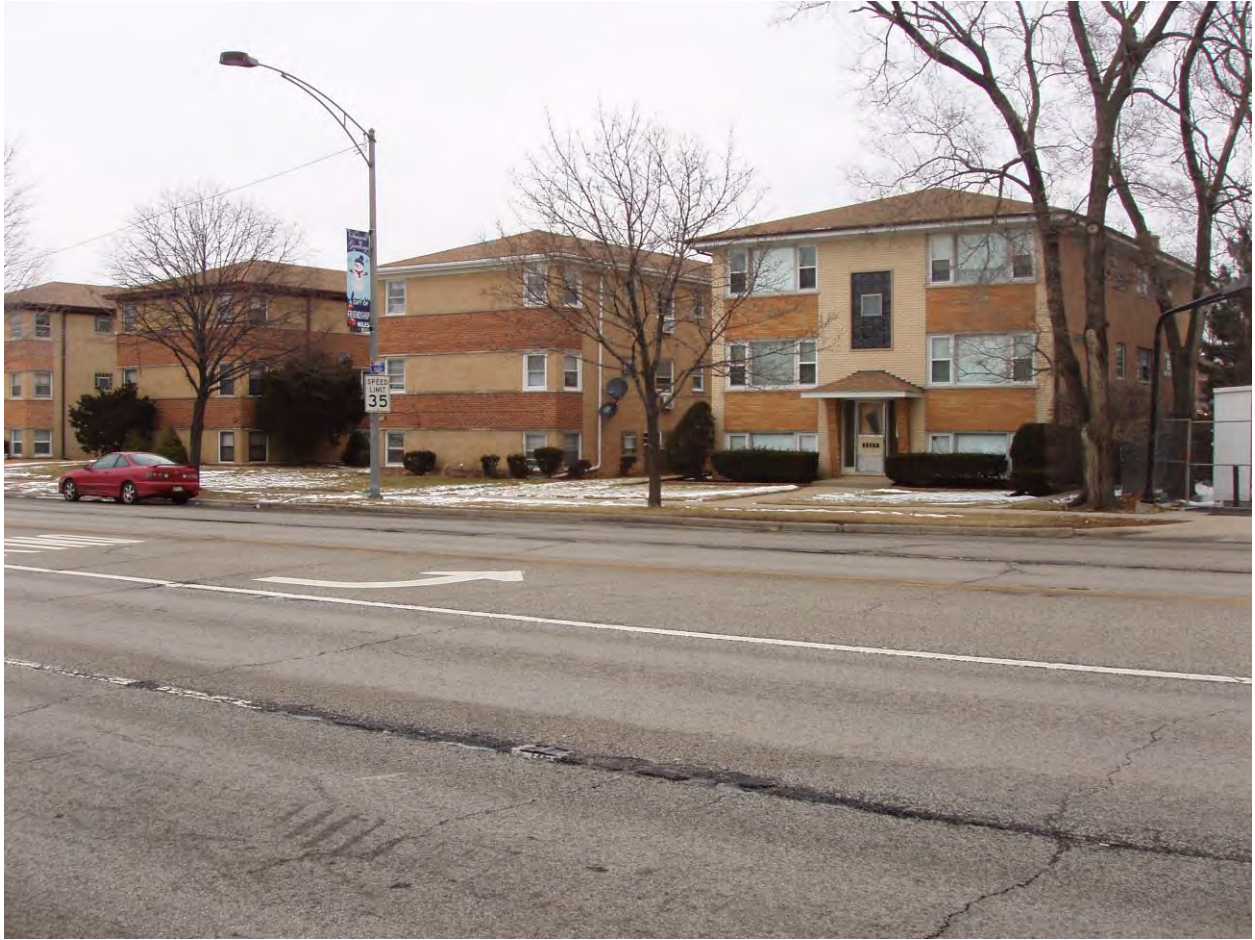
View to 8409 N. Milwaukee Avenue from Proposed Station Location
