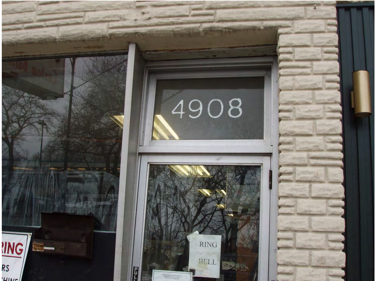
Building 030 - 4908 N. Milwaukee Avenue - Close-Up
