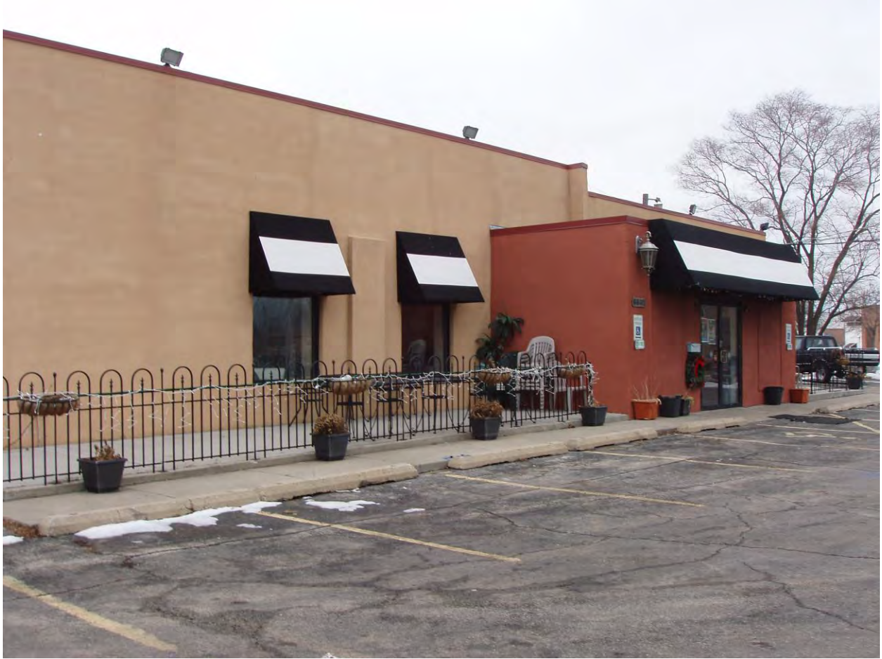
8801 N. Milwaukee Avenue - View to Northeast
