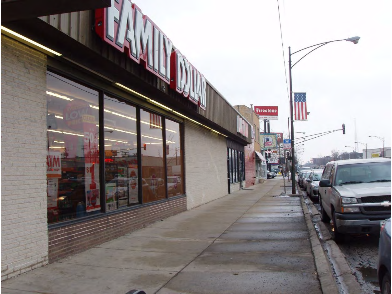
View of Farragut Avenue to Foster Avenue
