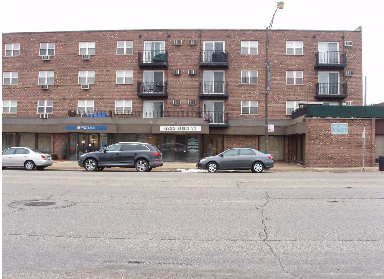
6333 N. Milwaukee Avenue View to Building from Proposed Station Location
