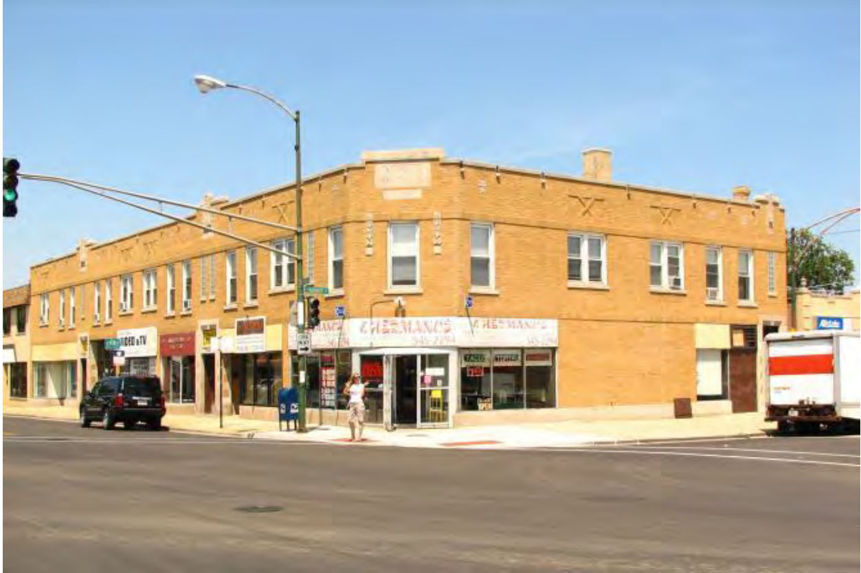
Building 021 - 5283 N. Central Avenue
