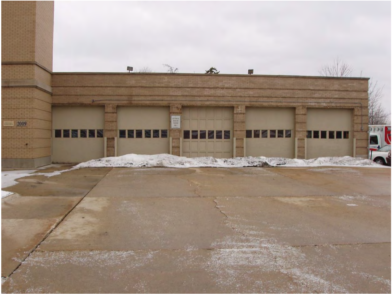
Garages on 8970 N. Milwaukee Avenue (Building 009)
