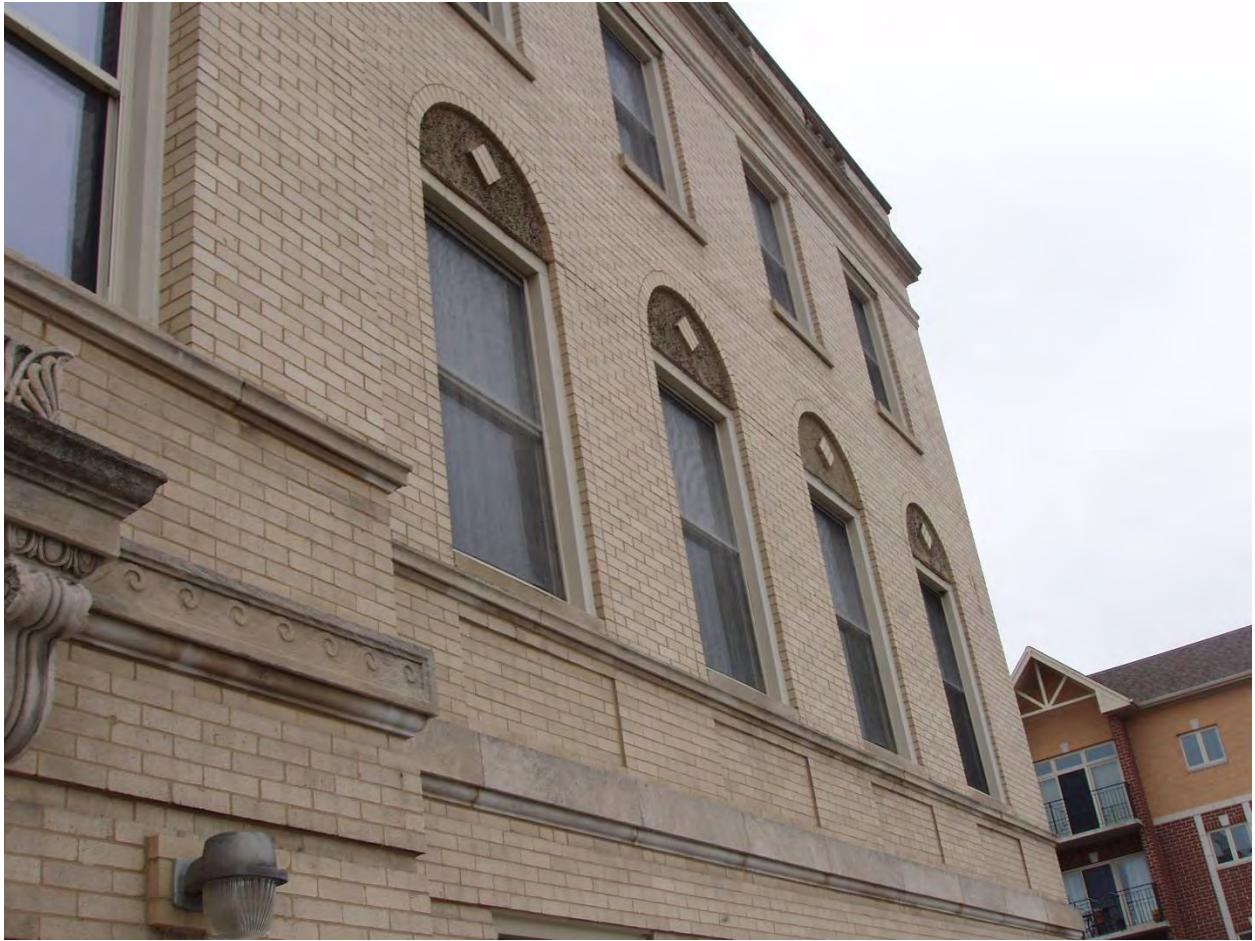
Windows on 8970 N. Milwaukee Avenue (Building 009)
