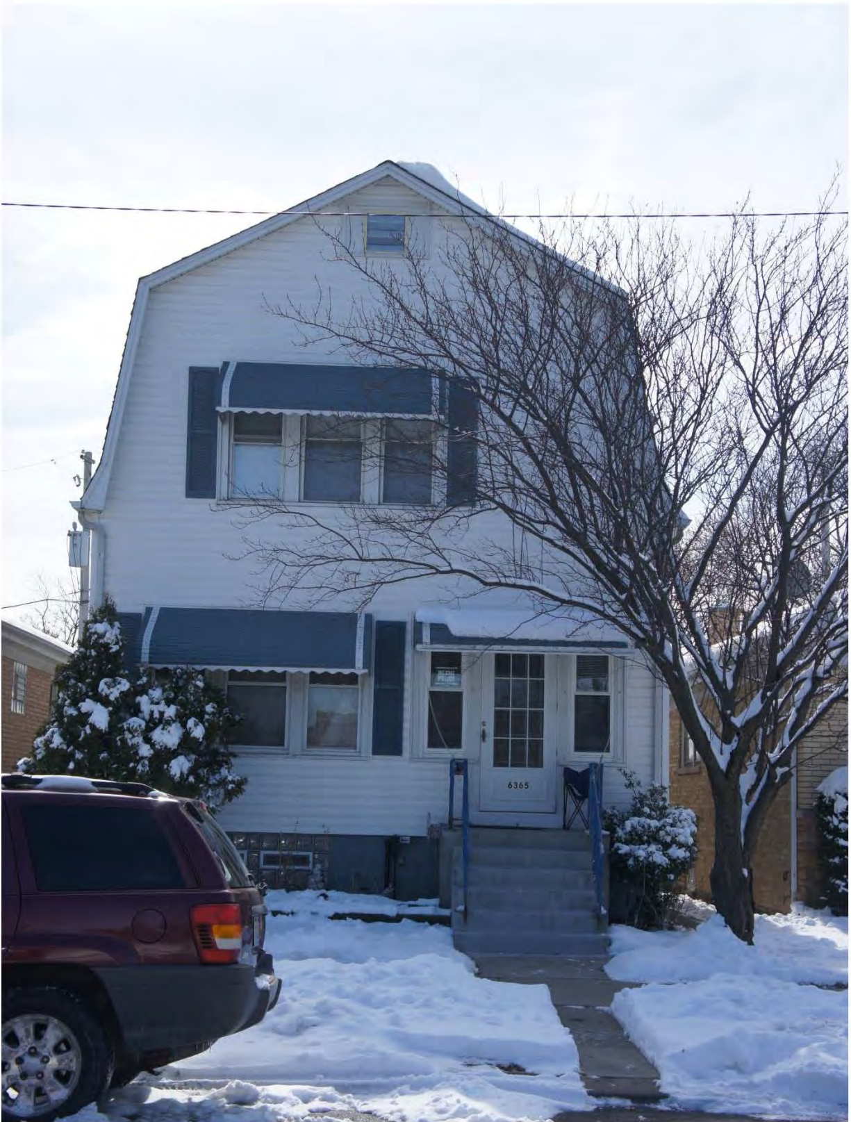
Building 008 - 6365 W. Haft Street
