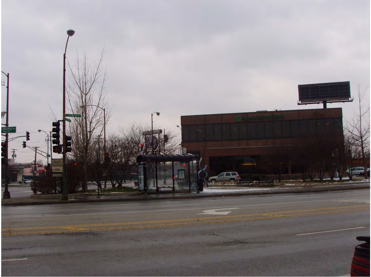
View of Proposed Station Location from 5251 N. Milwaukee Avenue (Property 039)
