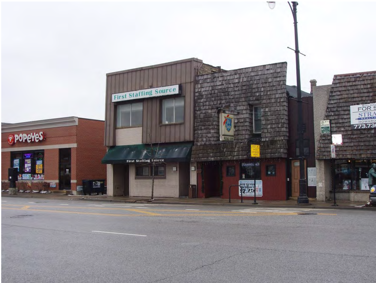
Buildings 002 and 006 - View to 4872 and 4874 N. Milwaukee Avenue from Jefferson Park Station
