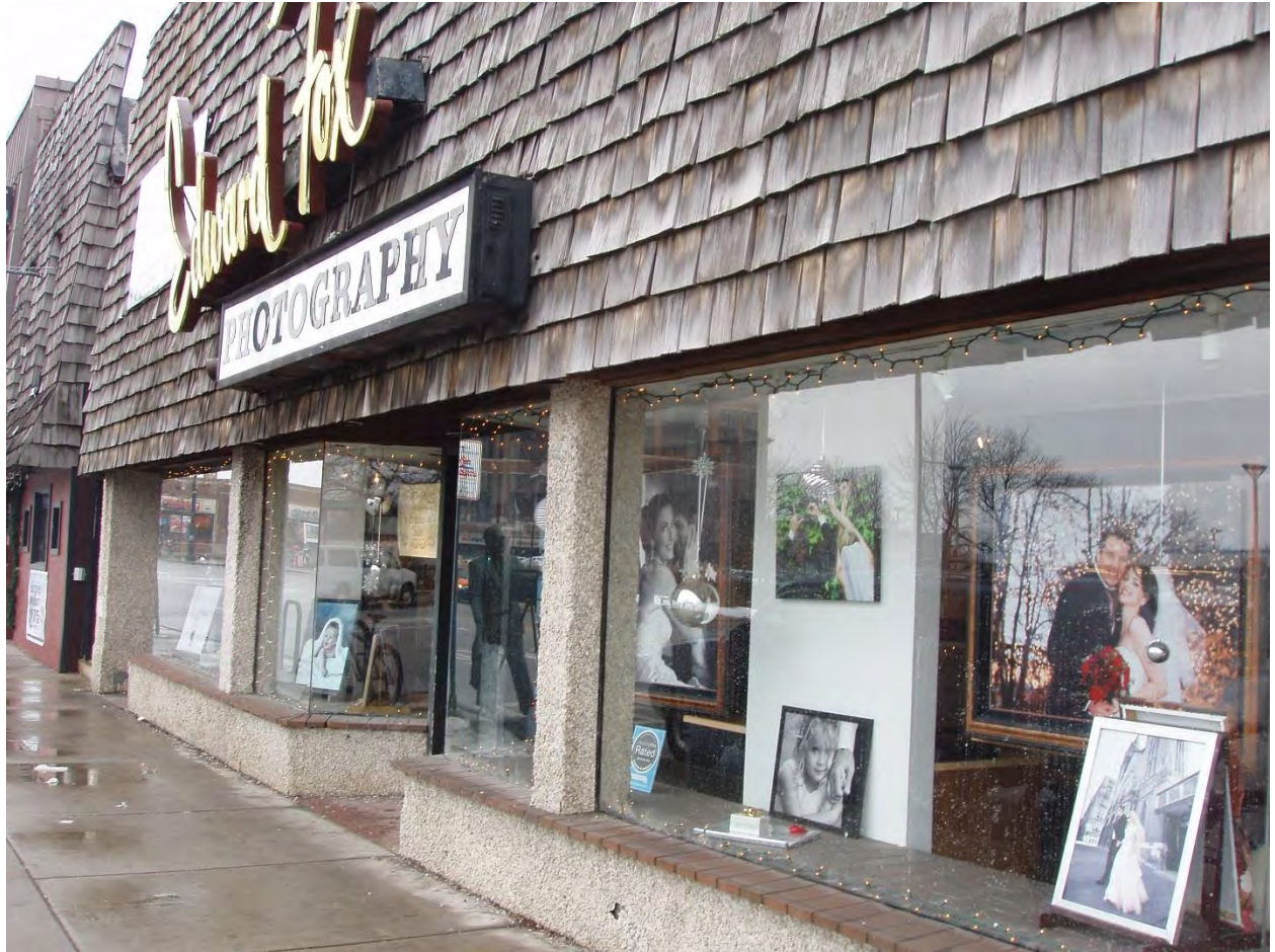
Building 011 - Edward Fox Photography - 4904 Milwaukee Avenue
