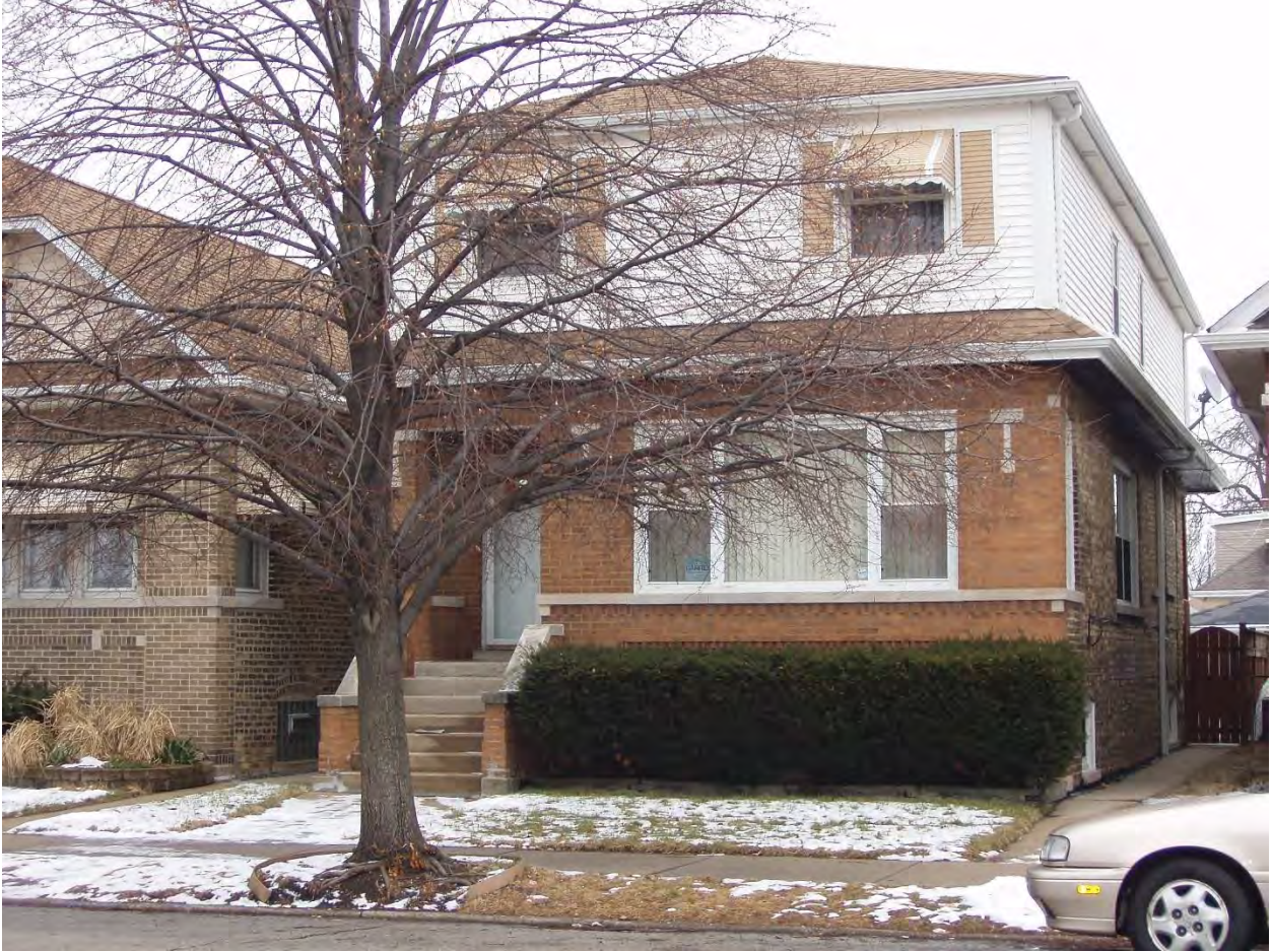
5847 N. Austin Avenue Noted as 5849 N. Austin in Assessor Records
