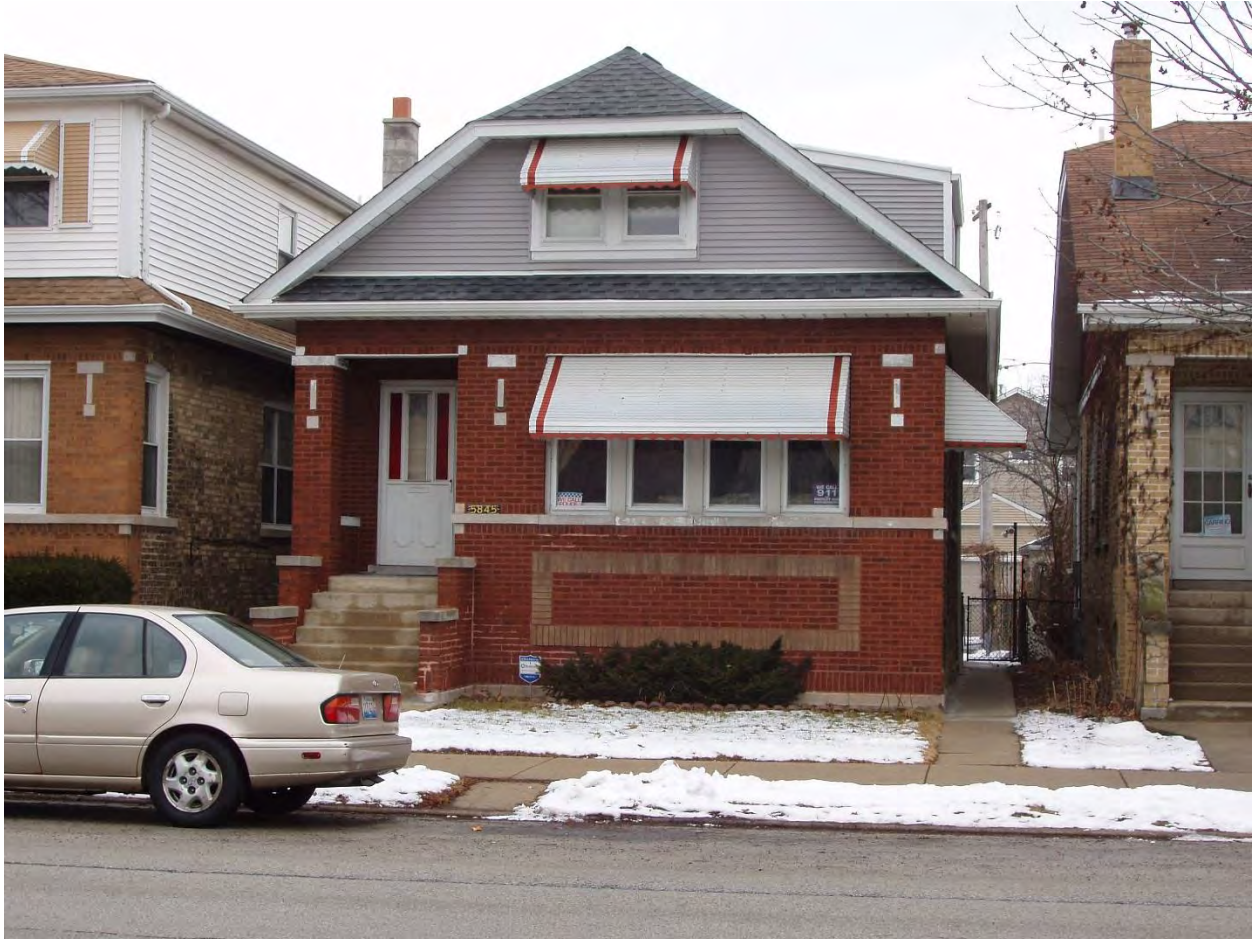
Building 025 - 5845 N. Austin Avenue
