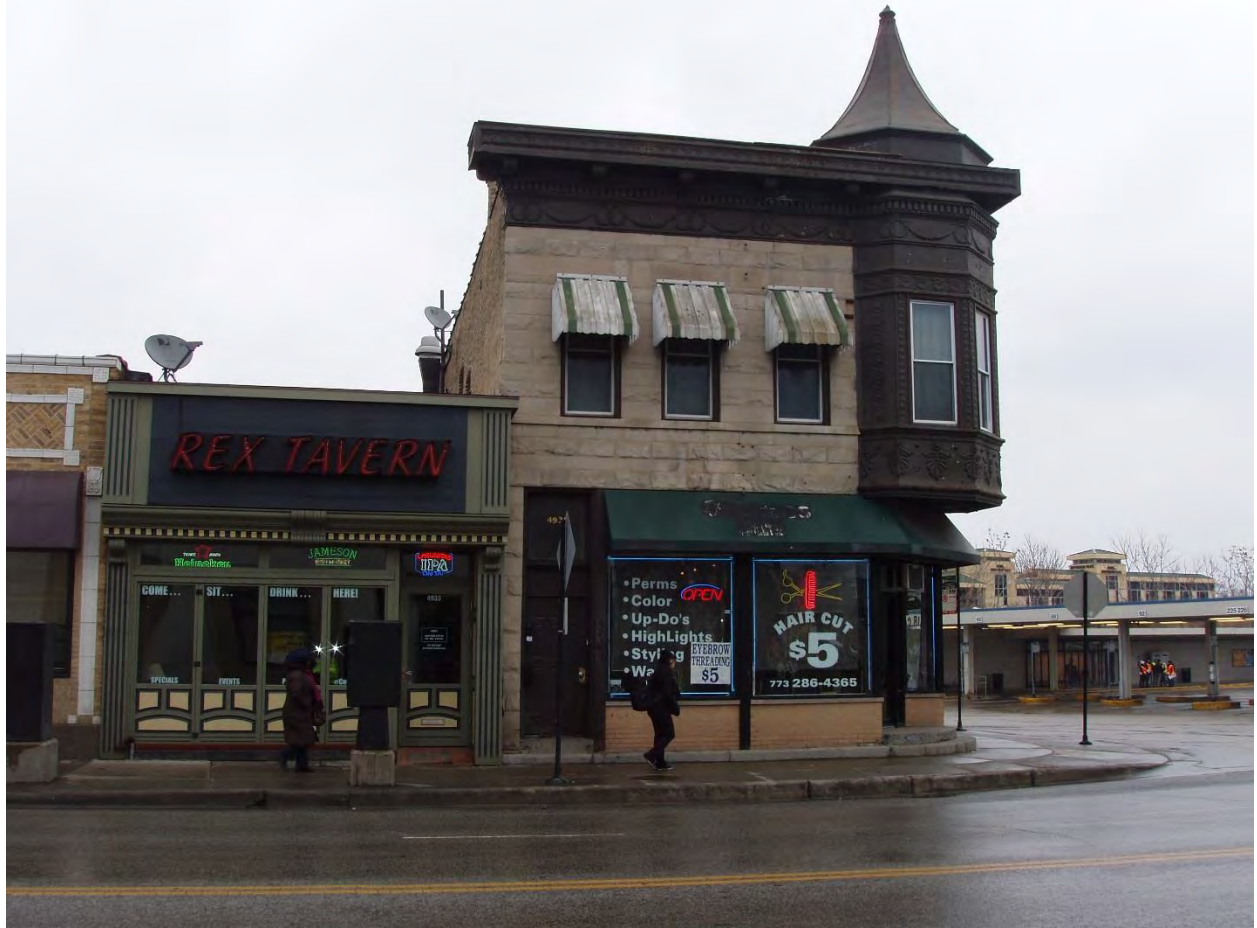
Buildings 004 and 020 - View to 4931 and 4933 N. Milwaukee Avenue
