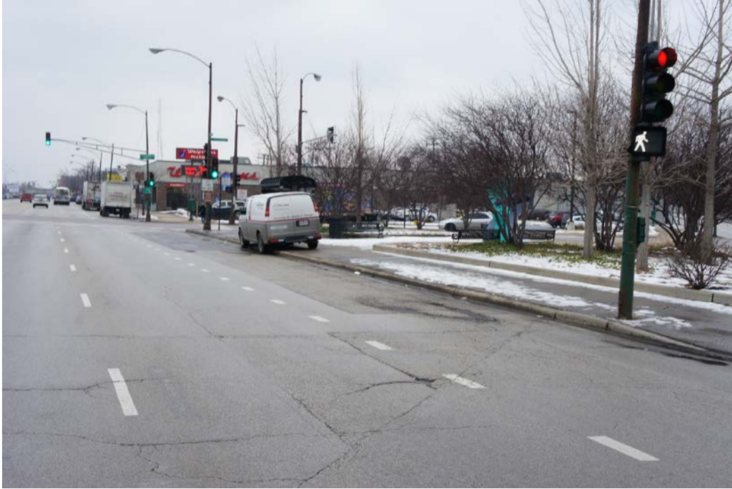
Photo 2: View of proposed southbound station location, on this landscaped triangular-shaped parcel, looking south. The existing southbound station is located behind the maintenance van in this photo.
