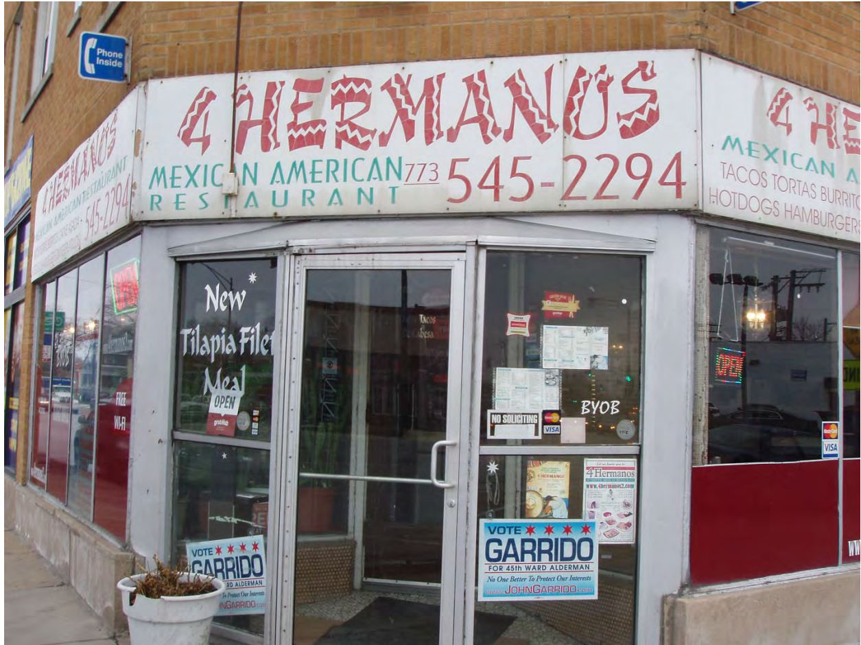
Building 021 - 5283 N. Central Avenue View from Northeast
