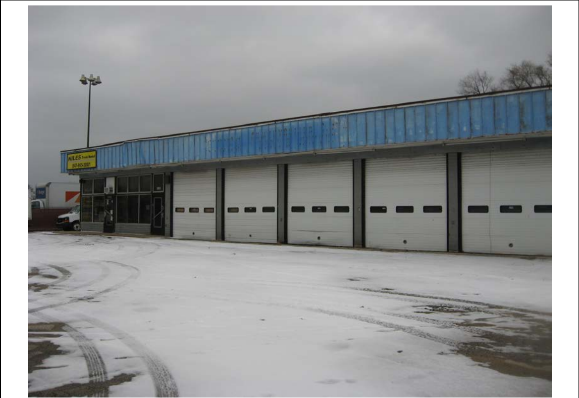
Photo 2: The Niles Truck Rental property appears to be a former car repair/gas station facility, looking east.
