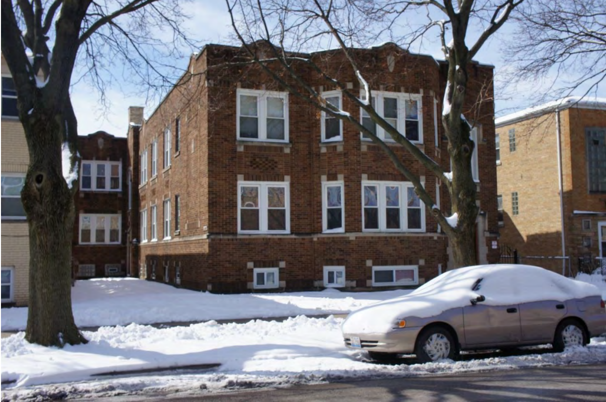
Building 028 - 6005 W. Ardmore Avenue
