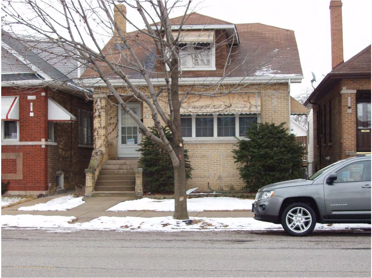
Building 024 - 5843 N. Austin Avenue
