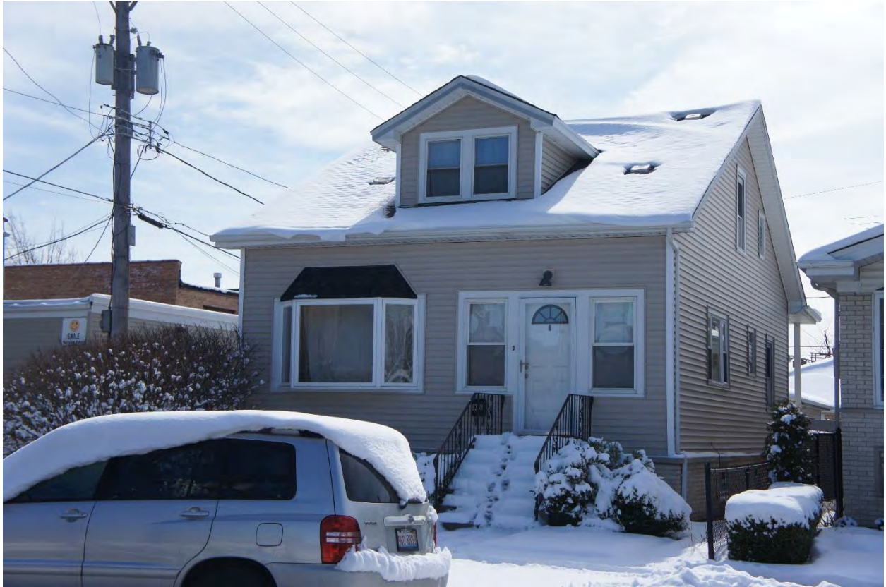
Building 007 - 6359 W. Haft Street
