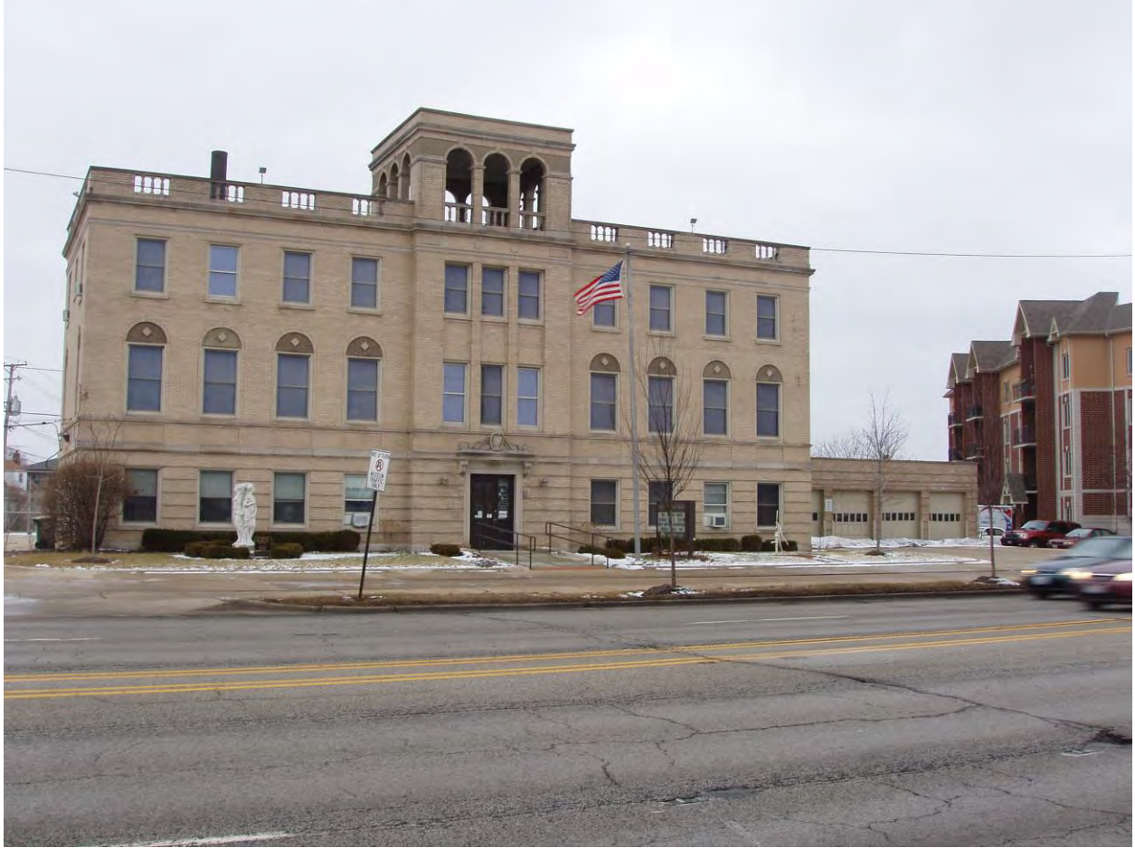
View to Cook County Sheriff Building - 8970 N. Milwaukee Avenue (Building 009)
