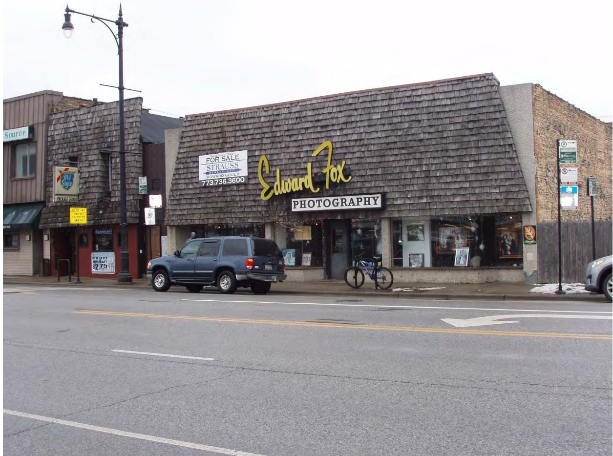
View to Edward Fox Photography (4904 Milwaukee Avenue [Building 011]) from Jefferson Park Station
