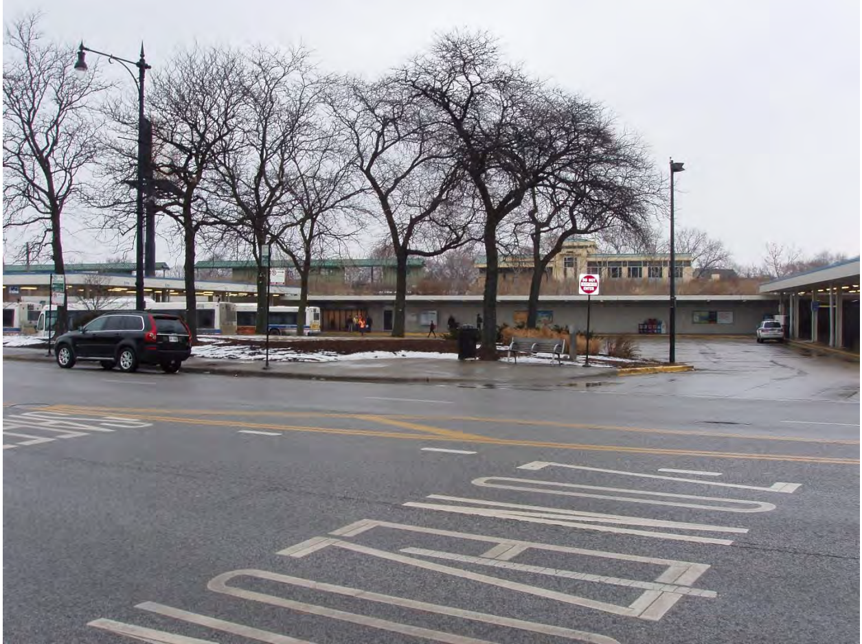
View to Jefferson Park Station from 4904 and 4908 N. Milwaukee Avenue (Buildings 011 and 030)
