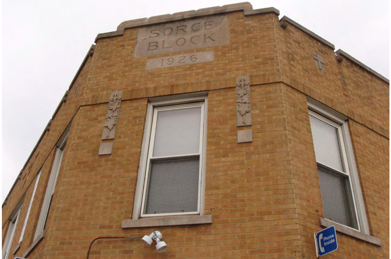
Building 021- 5283 N. Central Avenue
