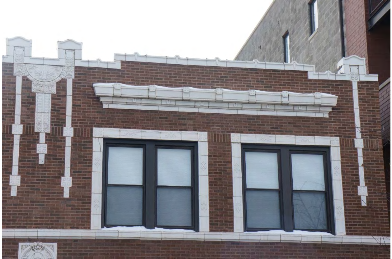
Building 019 - 4958 N. Milwaukee Avenue (2 nd Story Windows)
