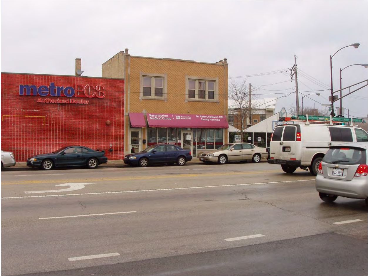
5249 and 5251 N. Milwaukee Avenue (Property 039) View to Buildings from Proposed Station Location
