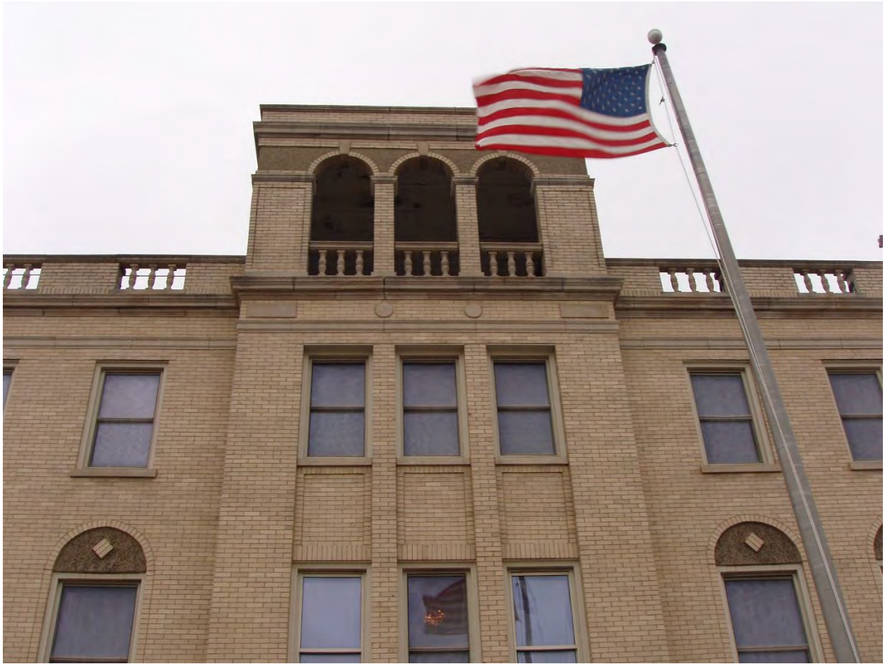
Close-Up of Roof Detail on the Cook County Sheriff Building (Building 009)
