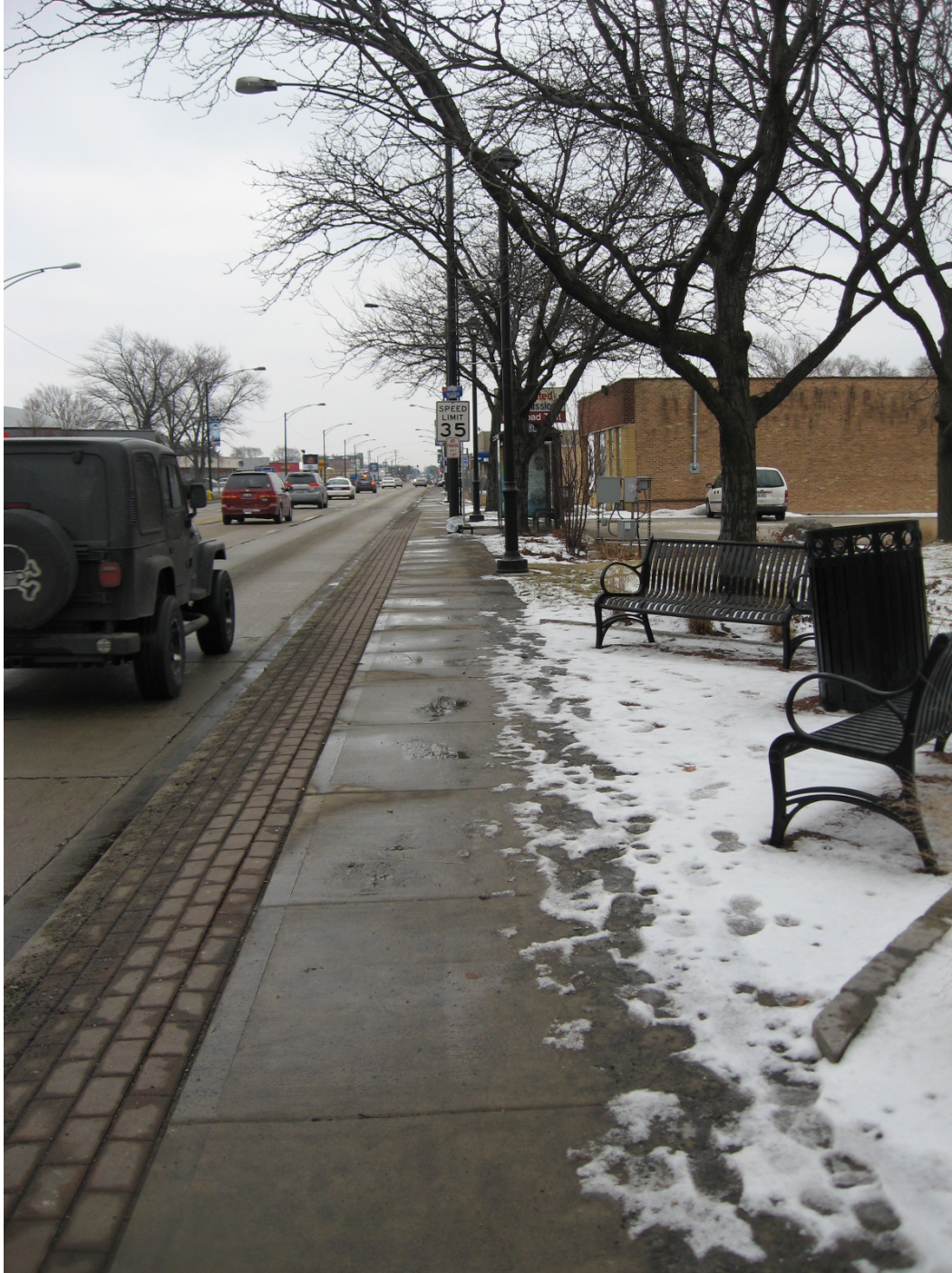
Photo 3: View of the proposed location for the southbound Harlem/Howard Station, looking southeast. Several electrical panels are visible near the existing PACE stop.
