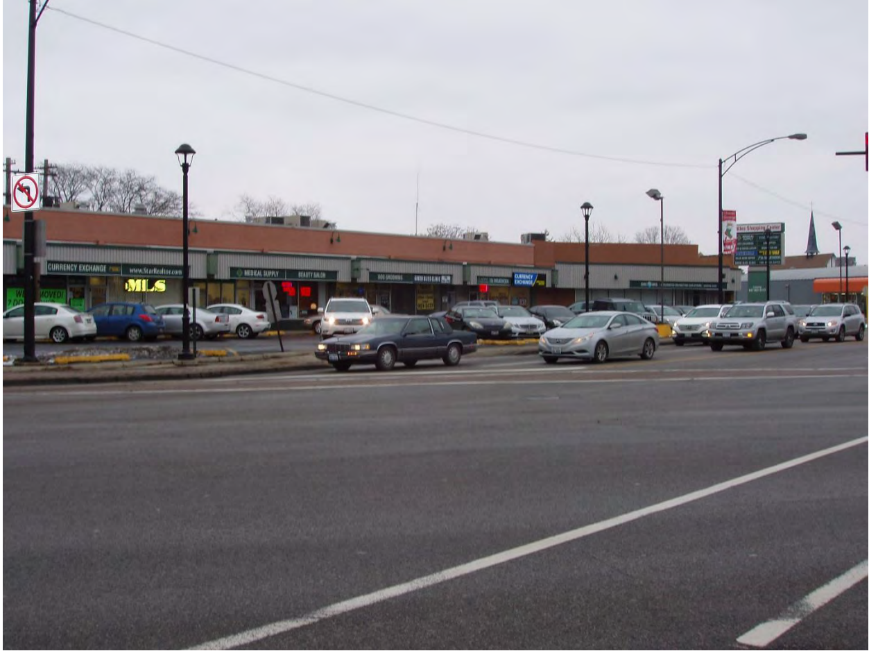
Niles Shopping Center Southeast Corner of Milwaukee Avenue and Harlem Avenue
