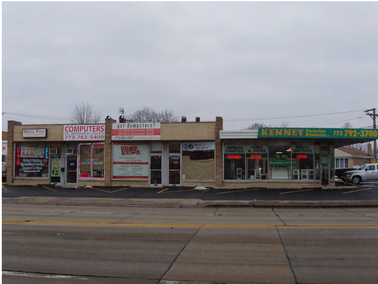
7570 to 7560 N. Milwaukee Avenue View to Building from Proposed Station Location
