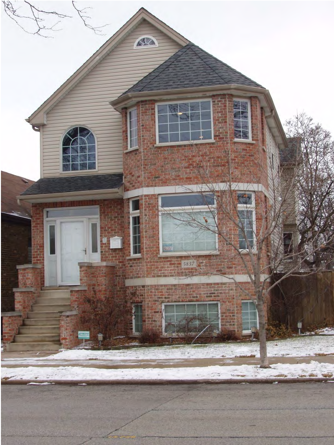
Building 001 - 5837 N. Austin Avenue
