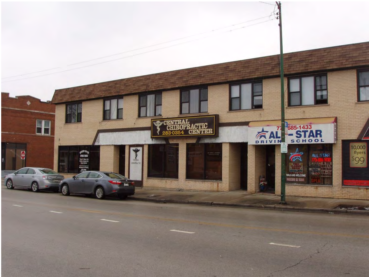
5257 to 5265 Central Avenue Noted as 5285 to 5291 N. Central Avenue within the Assessor Records
