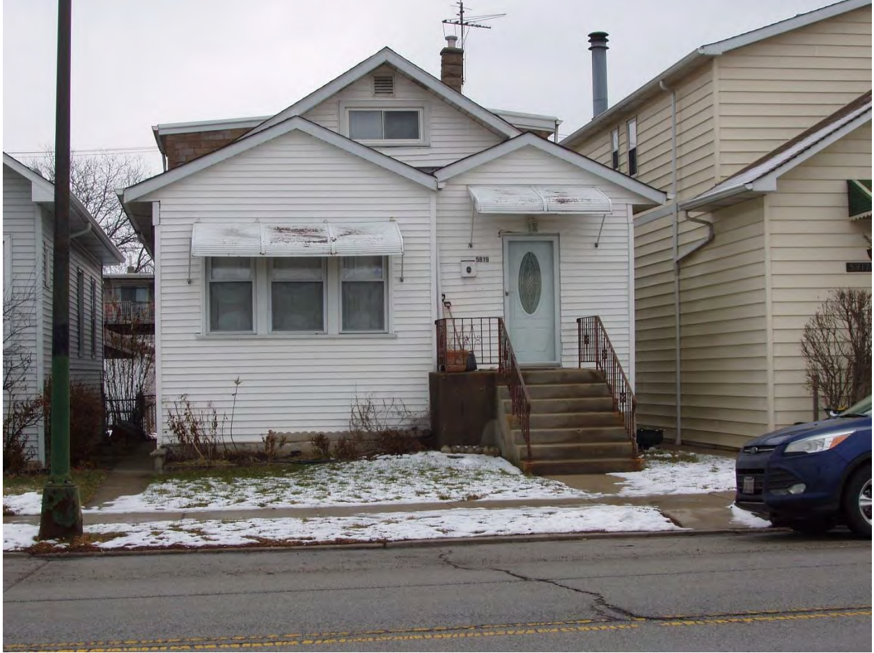
Building 015 - 5819 N. Austin Avenue
