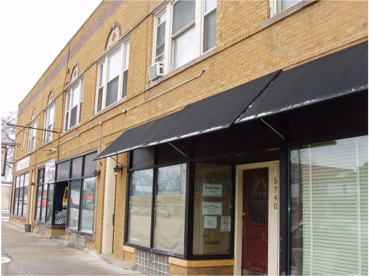
5740 N. Milwaukee Avenue to End of Block (View to South)
