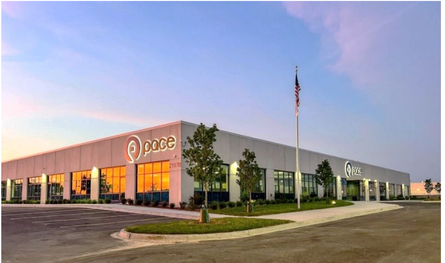
Photo: South Campus Administrative Building and Acceptance Facility, Markham, IL
